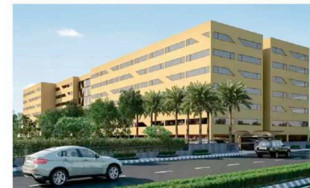
Indraprasth Business Park (Corporate Offices)
