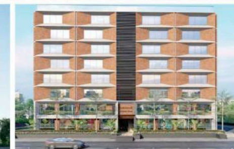
Indraprasth Business House (Showrooms & Offices)
